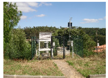
Met station near dam
